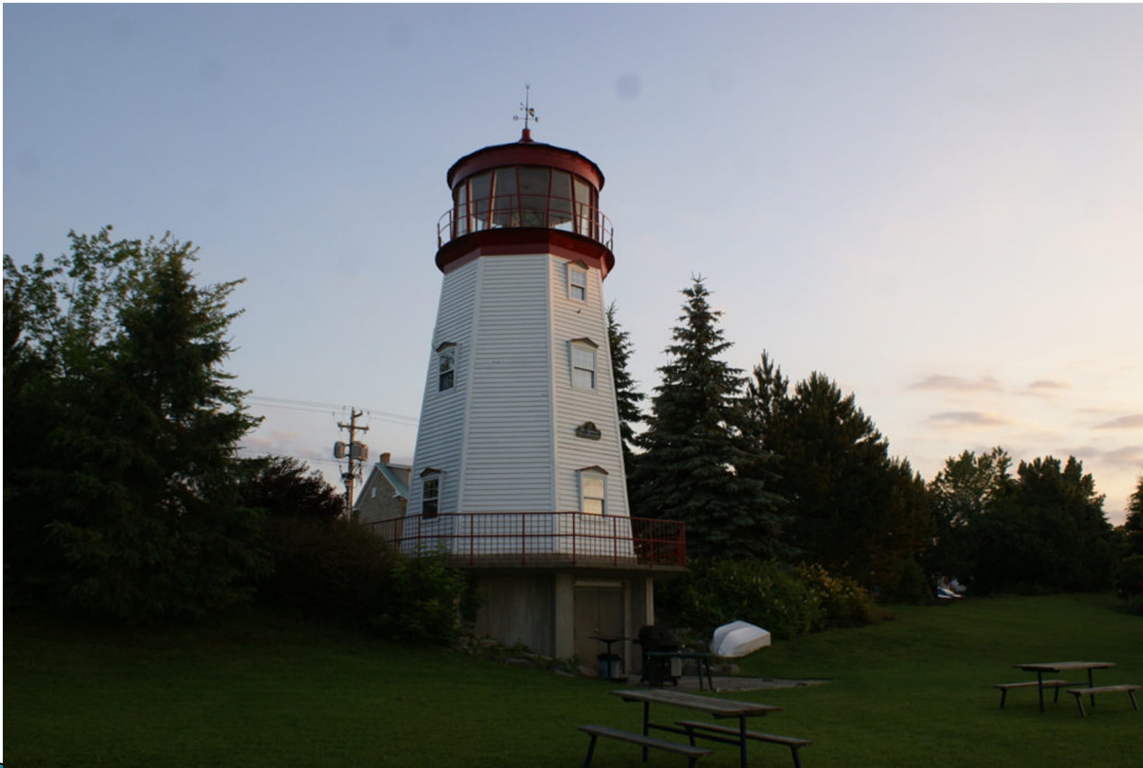
Can-Ont-Prescott Visitor's Center
